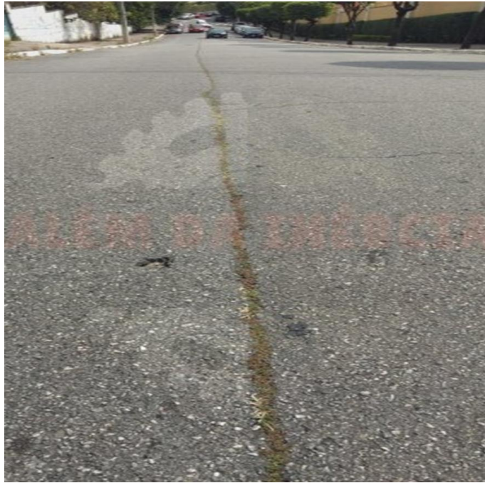
Figura 19 - Bombeo (Pumping and Water Bleeding). Fuente: Autor (2018)
