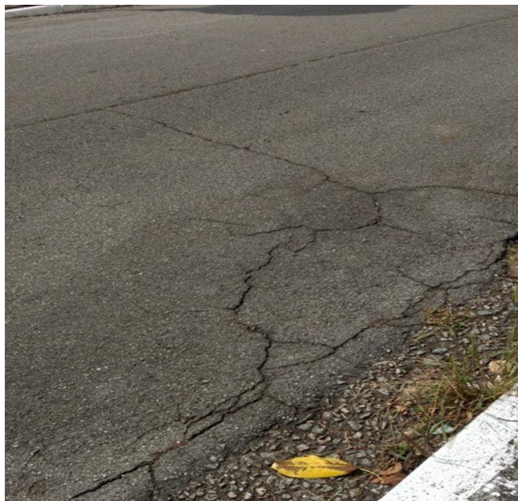
Figure 21 - Edge Cracking. Source: Author (2018)
