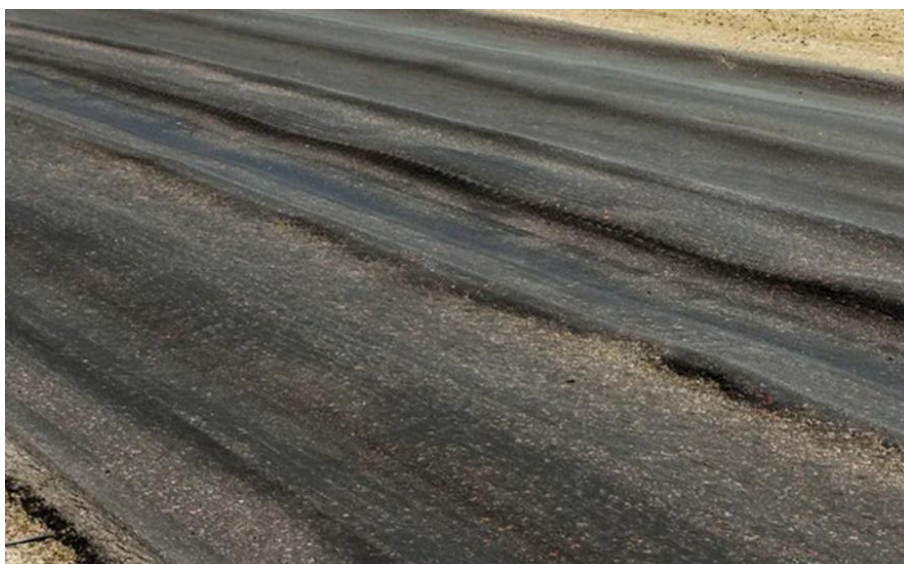
Figure 23 - Deformations or ripples caused by the passage of very heavy vehicles and/or poor quality of the applied base
