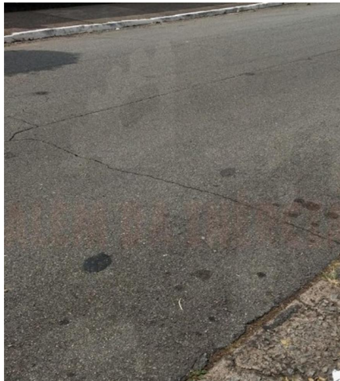
Figure 18 - Transverse Cracking. Source: Author (2018)
