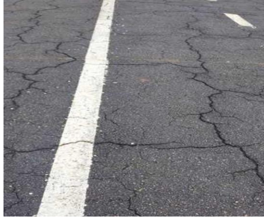
Figure 10 - Block cracking. Source: Author (2018)
