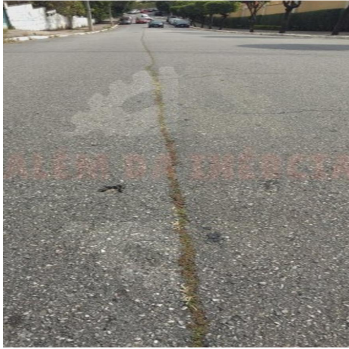
Figure 19 - Pumping and Water Bleeding. Source: Author (2018)
