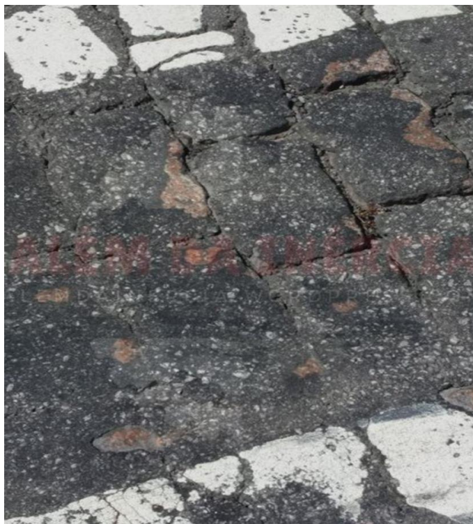
Figure 16 - Reflection Cracking. Source: Author (2018)
