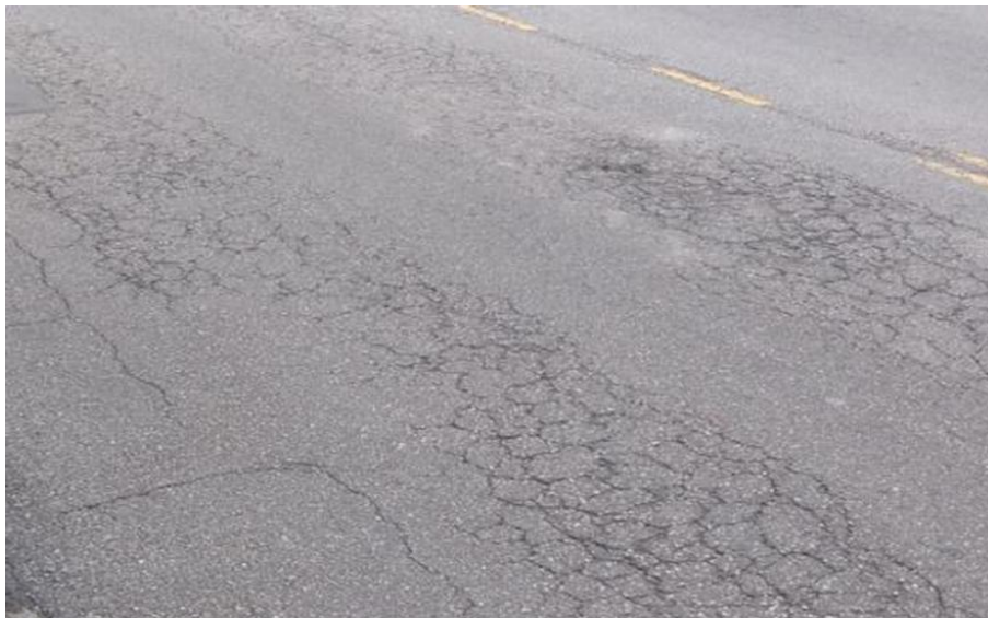
Figure 9 - Permanent Deformation (Rutting) and Fatigue Cracking in the wheel track.
