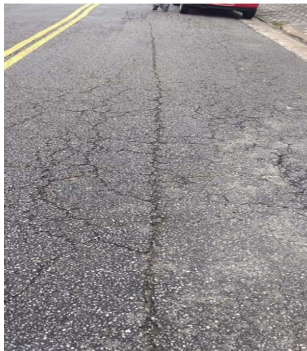
Figure 11 - Longitudinal Cracking. Source: Author (2017)
