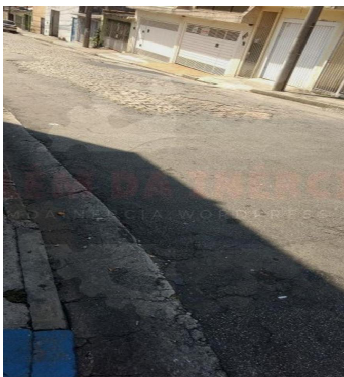
Figure 17 - Lack of adhesion on cobblestones. Source: Author (2018)
