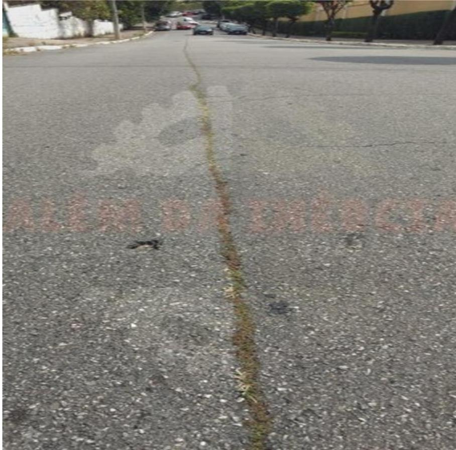
Figura 16 - Bombeamento (Pumping and Water Bleeding). Fonte: Autor (2018)
